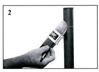
Place the PipeMaster on one of the stubs with the alignment marker over the centerline. Adjust the pins to fit the joint and mark the location of the plastic housing on the stub.
